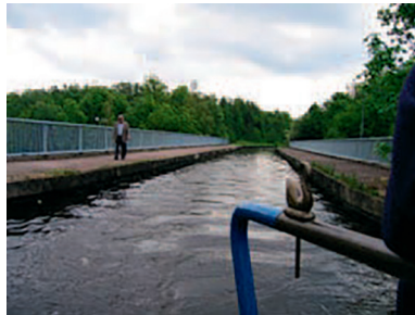
6. Burnley. The Leeds/Liverpool Canal passing over a four-lane motorway.
