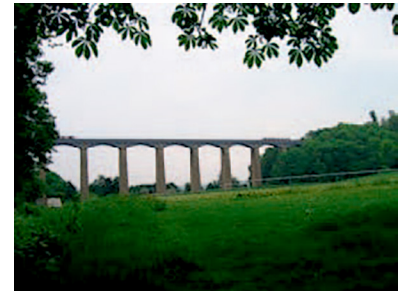
8. Wales, the Llangollen Canal, the Pontcysyllte Aqueduct. Distant View.
