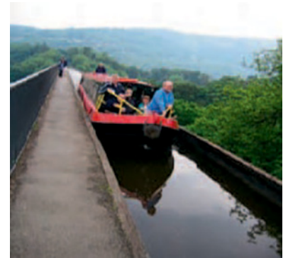
9. Wales, the Llangollen Canal, the Pontcysyllte Aqueduct. View of Telford and Jessop's cast iron trough.
