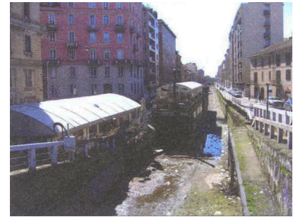
Pavia Canal today near the Port of Ticino, rotting boats in foreground
